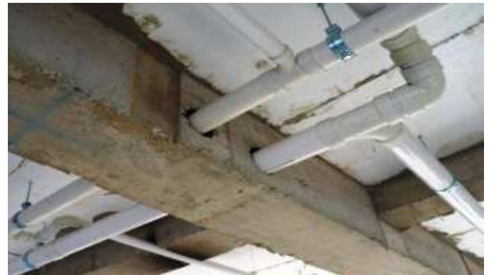
Fig -1: Water pipe passing through straight beam
