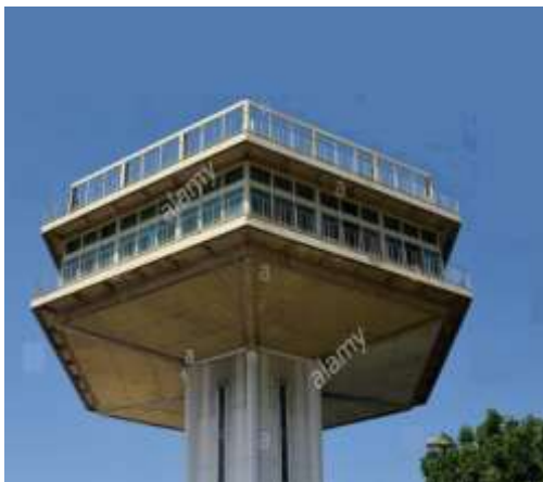
Fig -3: Watch towers in hexagonal beams shape
