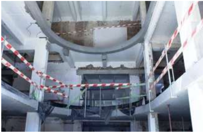
Fig -2: Curved beam of a building under construction
