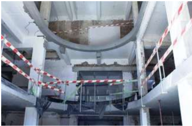
Fig -2: Curved beam of a building under construction
