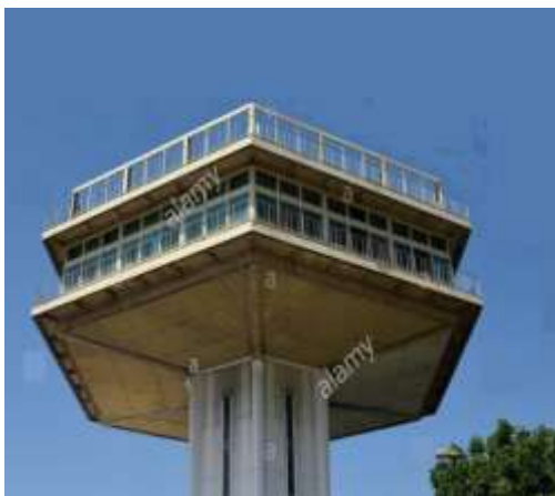
Fig -3: Watch towers in hexagonal beams shape
