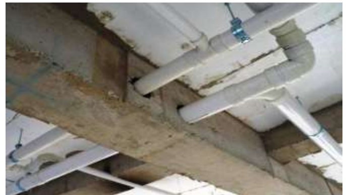
Fig -1: Water pipe passing through straight beam
