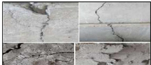
Fig.3 Structural cracks due to loading
