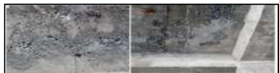
Fig.4Scaling of concrete
