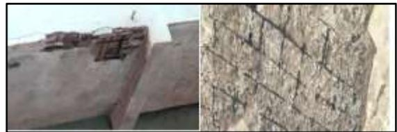
Fig.1 Spalling of concrete
