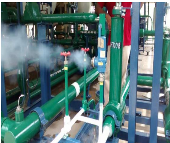
Fig 4.5: Cryogenic pressure relief valve
