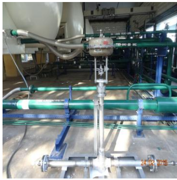
Fig 4.3: Cryogenic globe valve
