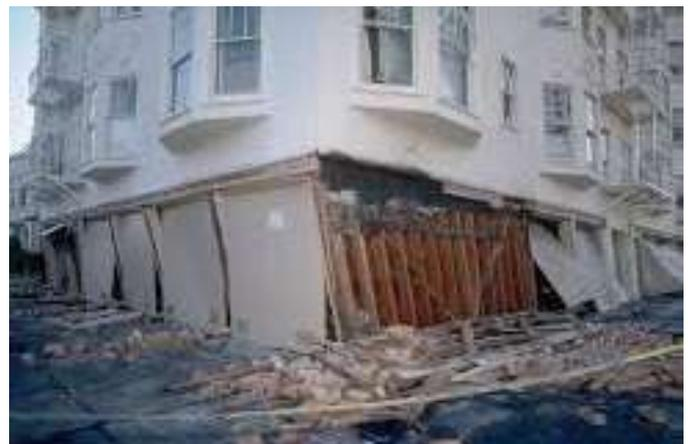
Fig-1: Typical open ground storey building
