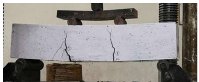
Fig. 4 cracking pattern of GFRP reinforced beam
