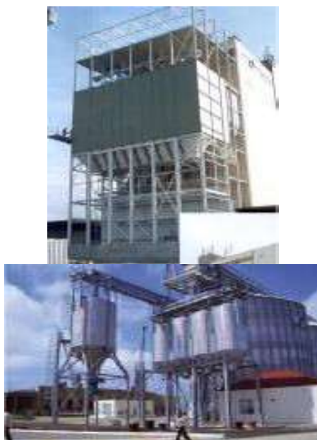
Fig. 2 Truck load silo
