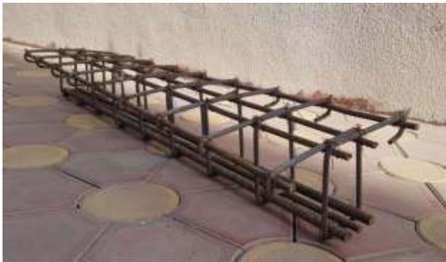
Fig -2: 3D View of Reinforcement Detailing of T- Beam
