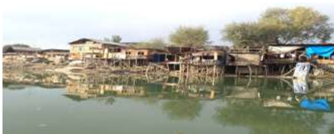
Encroachments along the river banks
