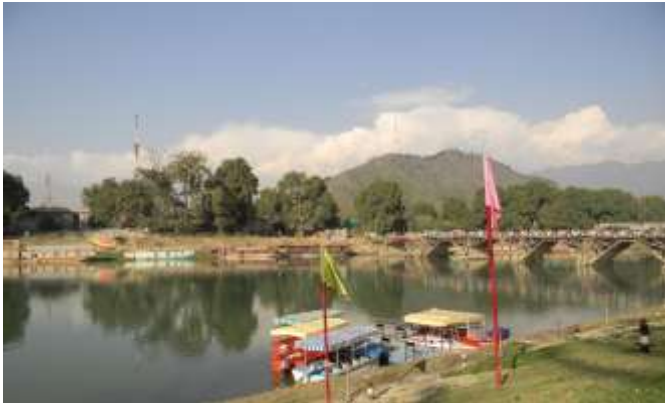
Terminal Station -Zero Bridge
