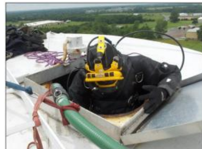
Fig-1: Conventional Water Tank Cleaning
