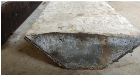
Fig-7: Failure of trapezoidal CSCC beam (side view)
