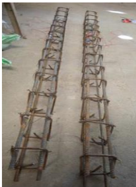
Fig -4: Reinforcement details of the beam
