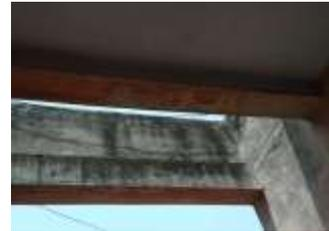
Fig -4: Flexural Cracks in Beam
