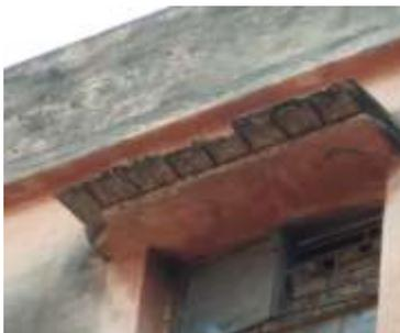
**Fig -9:** Failure of chajja
