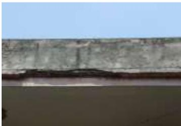
**Fig -8:** Deterioration of cover
