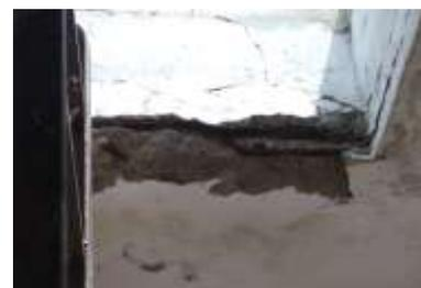
Fig -6: Spalling of concrete
