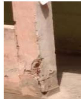
Fig -5: Cracks in Column
