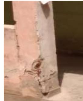
Fig -5: Cracks in Column
