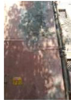
**Fig -10:** Flaking of plaster
