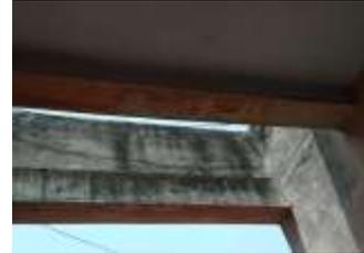
Fig -4: Flexural Cracks in Beam
