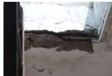
Fig -6: Spalling of concrete
