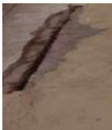
Fig -3: Reinforcement exposure
