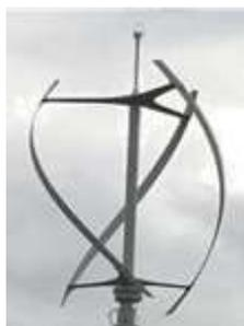
Fig-4: Gorlov Helical wind turbine
