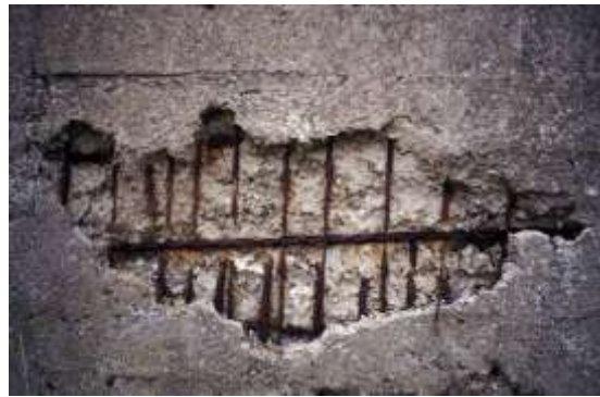
Fig-5: - Erosion Effect in R.C.C Slab
