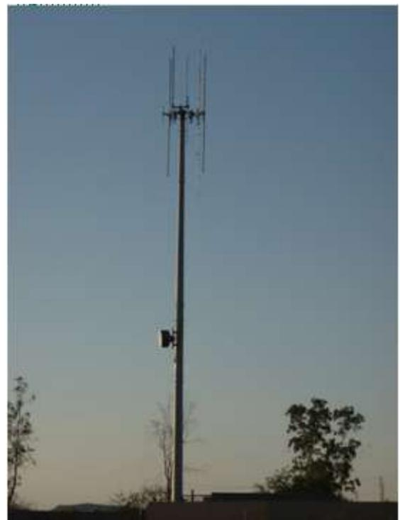
Below fig. Shows omnidirectional antenna
