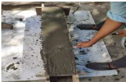
Figure -4 Casting of beam
