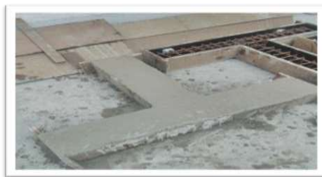
Fig 1 Reinforcement and casted Beam column joint
