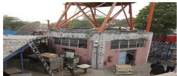
Fig: 1 View of Concrete Structure (ISRO, Delhi)
