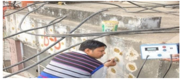
Fig: 3 UPV Test by Direct Method on RCC Beam
