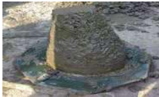
Fig- 2: Slump test
