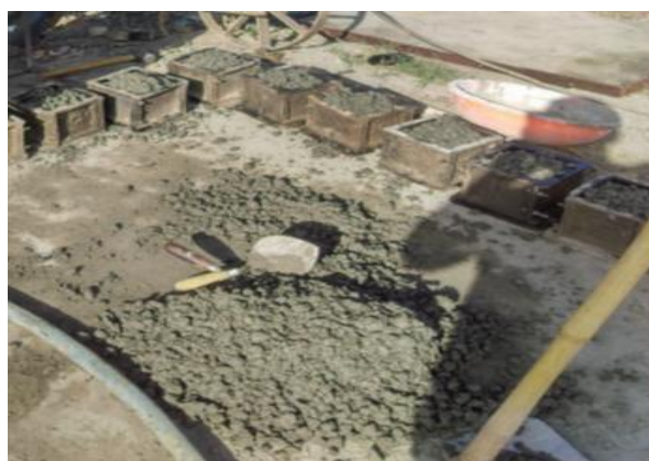
Figure no.1 Casting of cube at Site
