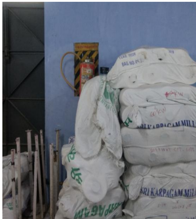
Figure 4.2 Extinguisher in unaccessible area
