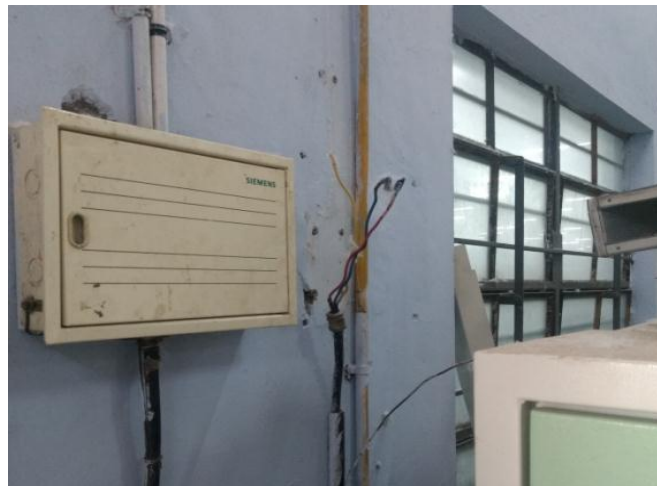
Figure 3.3 Improper wiring
