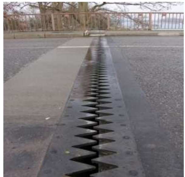
Fig -1: Expansion joints in bridge
