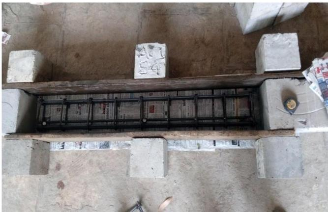
Fig 1: Placing of the cage in the mould
