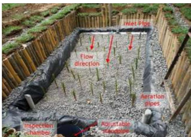
Figure 6: Process of treatment of waste by HSSF-CW method
