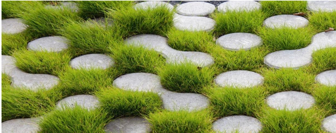
Figure : concrete grass pavers with lawn view.
