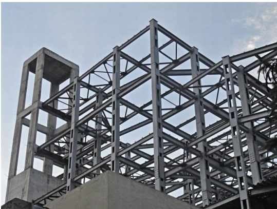
Fig 1.1: Steel building in India
