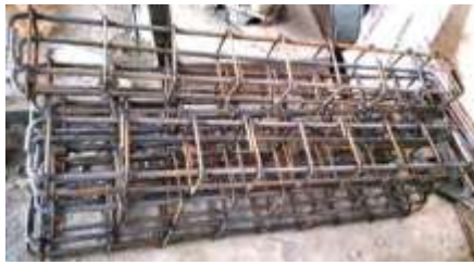
Fig -4: Reinforcement skeleton
