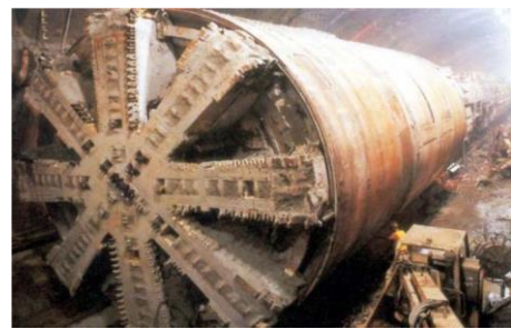
Fig -1: View of TBM
