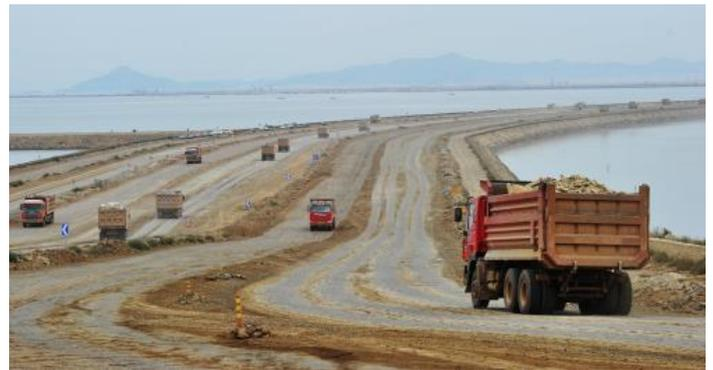
**Fig -9:** The trucks movement during the reclamation process Source: (Yin Pumin, 2014)
