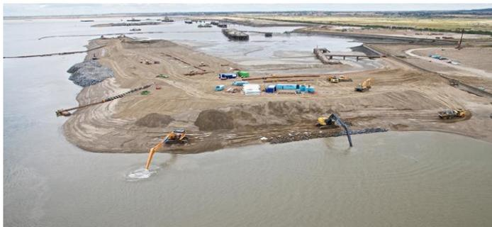
**Fig -7:** Illustration of the proposed reclaimed area location and method (source: DEME, 2014)
