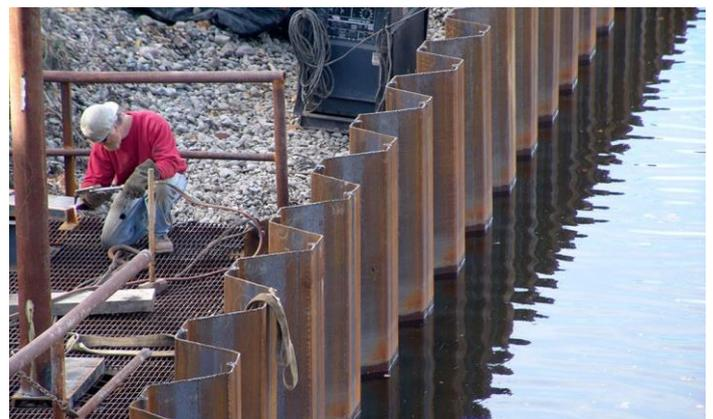
Fig -6: The proposed sheet pile section (PZC 28) (source: GERDAU, 2016)
