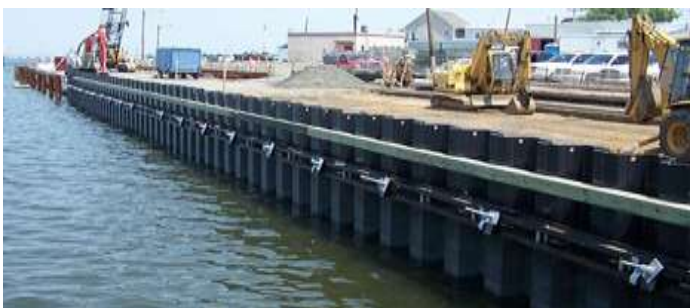
Fig -8: Installation of sheet piles (source: WIKI, 2016)
