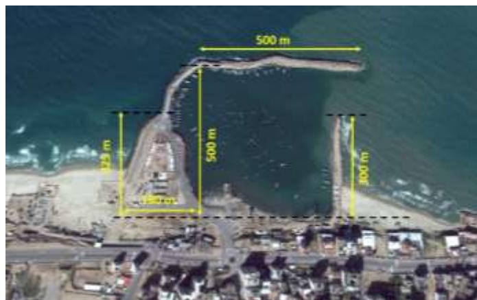
Fig -3: The existing Gaza fishing harbor (source: Google earth, 2016)
