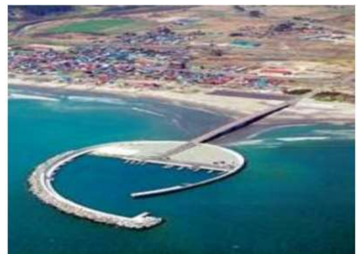
Fig -11: The general view of proposed reclamation and bridge installation (source: Xinhua, 2016)
