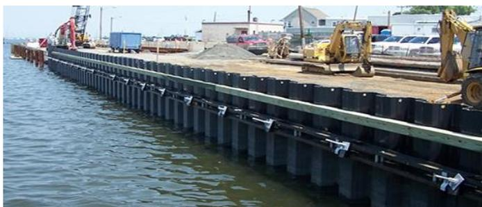
**Fig -8:** Installation of sheet piles (source: WIKI, 2016)
