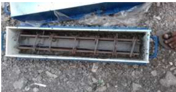
Fig -5: Casting of C-Channel GFRP beam
