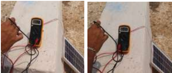
Fig -13: Current reading Fig -14: Voltage readings
