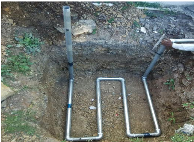
Fig. 1 Actual Set up Of EATHE system
