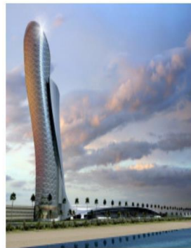
Fig. 3.7 Capital Gate Tower in Abu Dhabi
