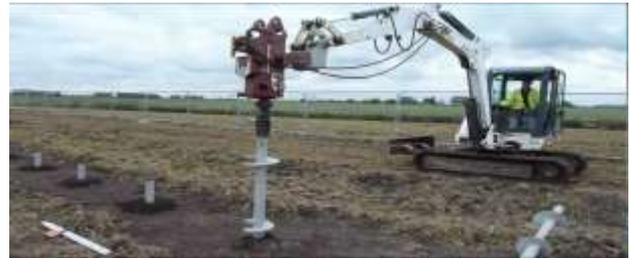
Fig-1.2: Installation of crew pile
