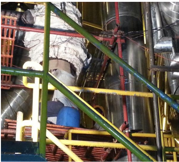
Fig 9: Insulated outer surface of the housing to minimize heat loss.
