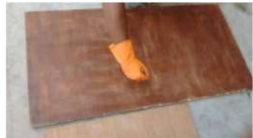
Fig 7: Application of Polyvinyl as releasing agent
