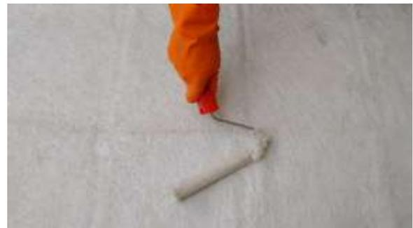
Fig 8: Removal of air bubbles using roller
