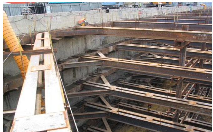
Fig -1: Strutted Diaphragm Wall
