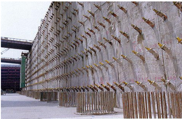
Fig -3: Anchored Diaphragm Wall
