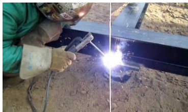
Fig.1.4 Weld connections
