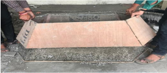
Fig -5: Demoulding
