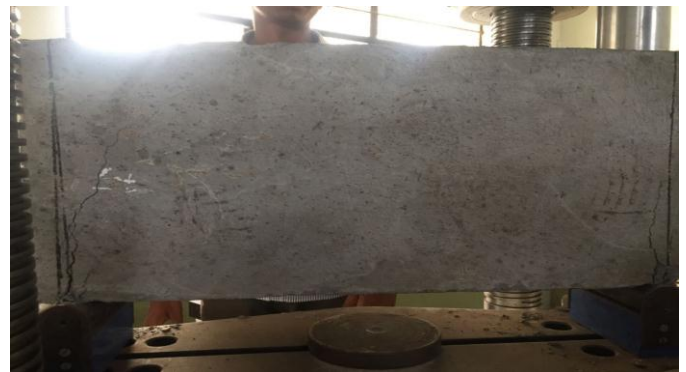
Shear failure and cracks on deep beam for Steel & BFRP
