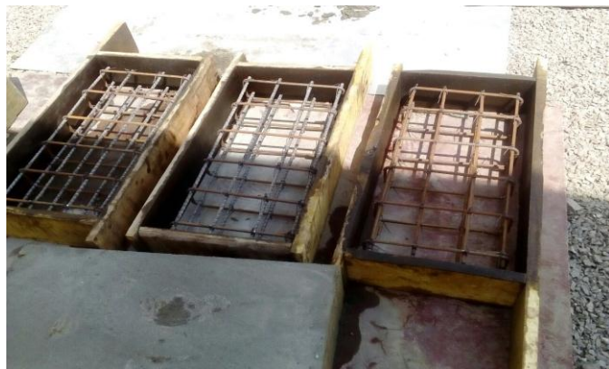
Placing of the cage in the mould
