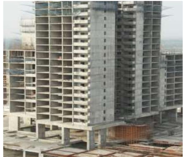
Fig 1. Transfer slab
