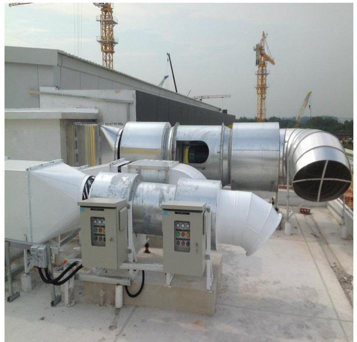
Fig: Exhaust air outlet in Industries.
