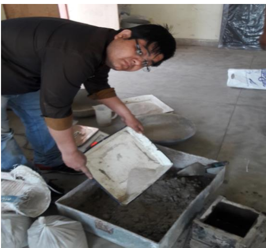
Picture 1: Mixing of Kota Stone Dust in the concrete
