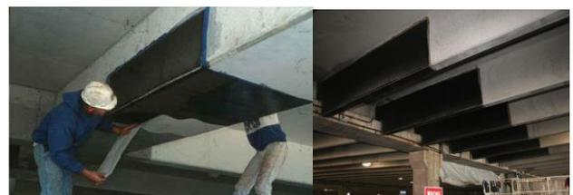
Fig 1.2; Strengthened beam with FRP laminates.
