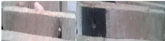
Fig 1.3 CFRP laminations inside and around the openings
