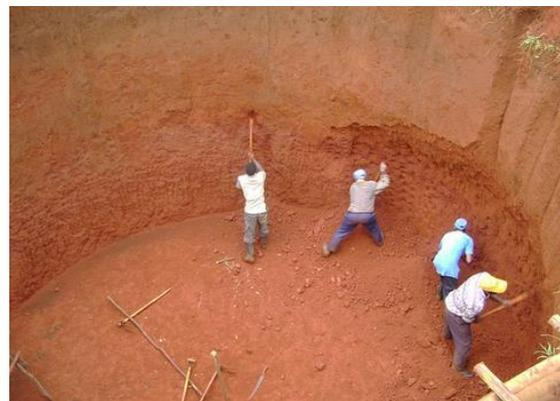
**Fig -4 Pit of Bio Gas chamber.**
