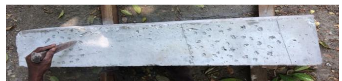
(c) Surface preparation
