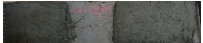
Fig -6: Failure pattern of UW-2B/M
