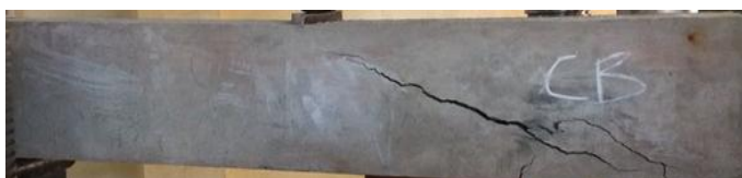
Fig -5: Failure pattern of control beam
