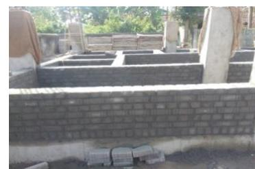
**Fig 3.8: Basement Wall Construction**
