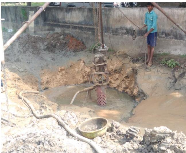
**Fig 3.9: Piles Foundation Trench**
