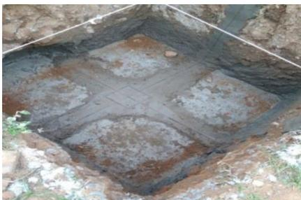
**Fig3.4: Column Center Line Marking**
