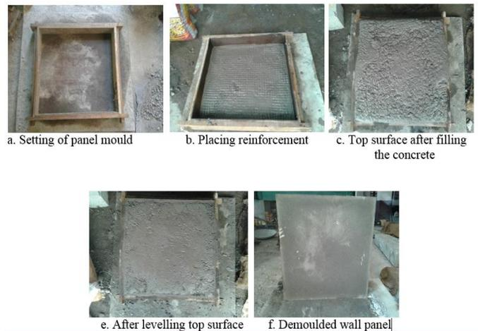
**Figure 3:** Typical views of sequences in casting of lightweight concrete wall panel
