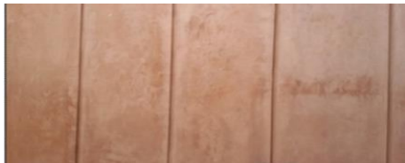
Fig.3. Color Lime Plaster
